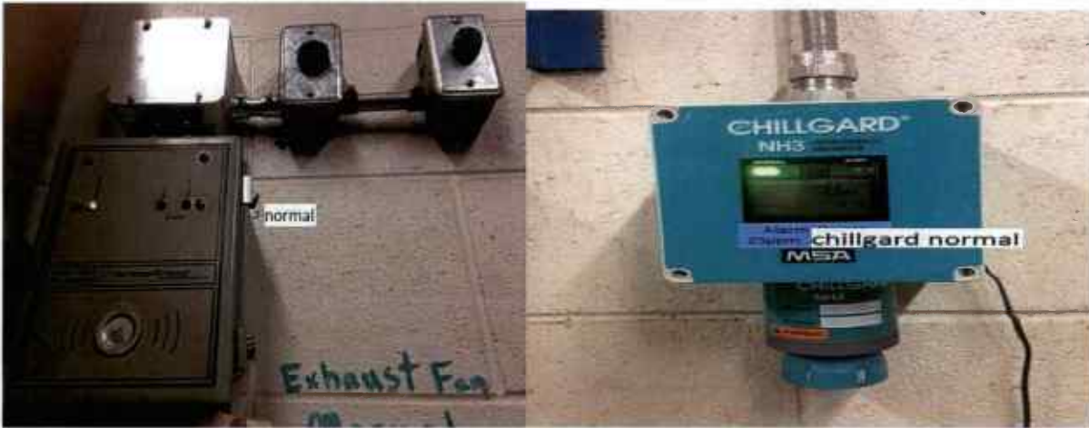
Armstrong – Normal Mode green light on Chillgard – Normal Mode – green light on
