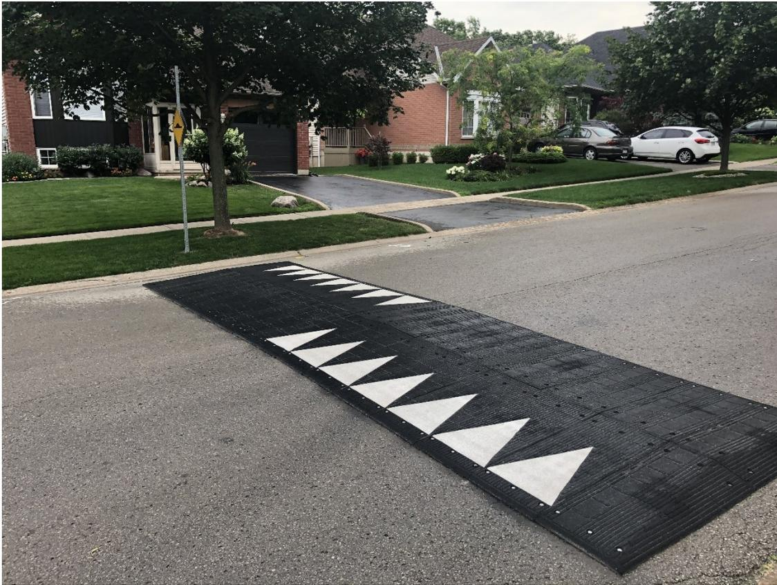
*Figure 2: Temporary Speed Hump Example*
