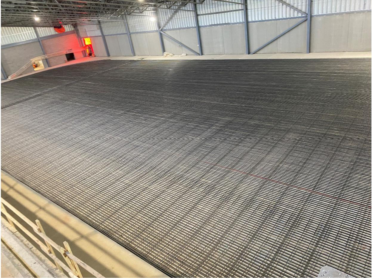
*Figure 14- Arena South - Cooling Lines - Prepour*
