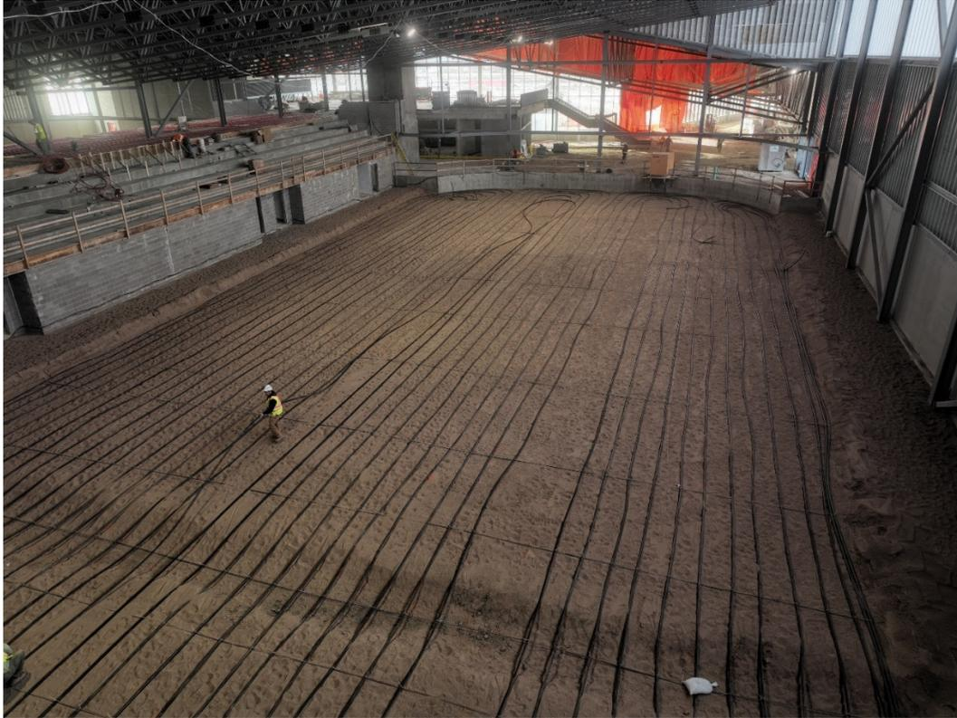
Figure 5 - North Arena - Heating Line Install
