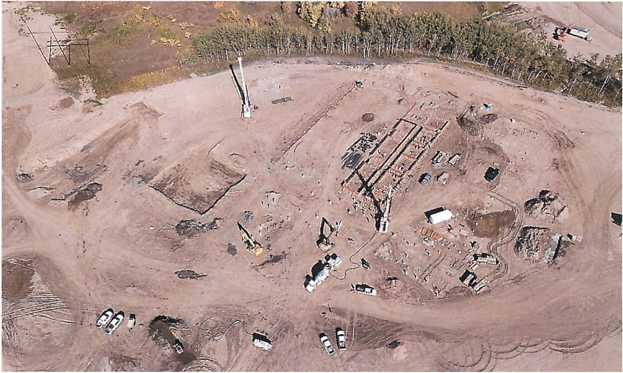
Overhead Drone photo as of September 28, 2022:
