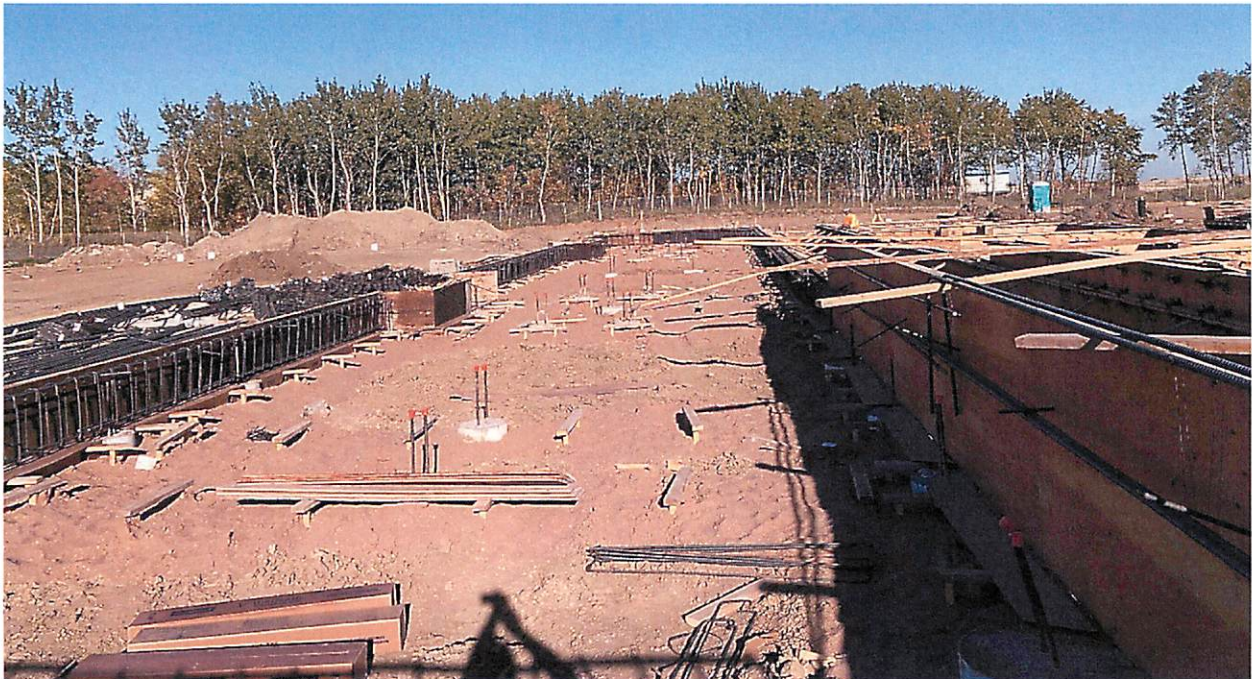
Forming and rebar installation to North Arenas dressing rooms:
