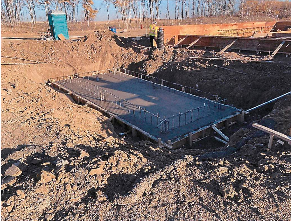
Snow melt pit formwork and hoarding:
