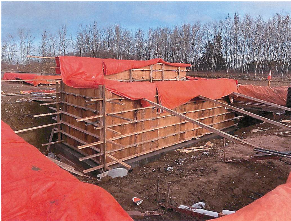
Snow melt pit formwork and hoarding:
