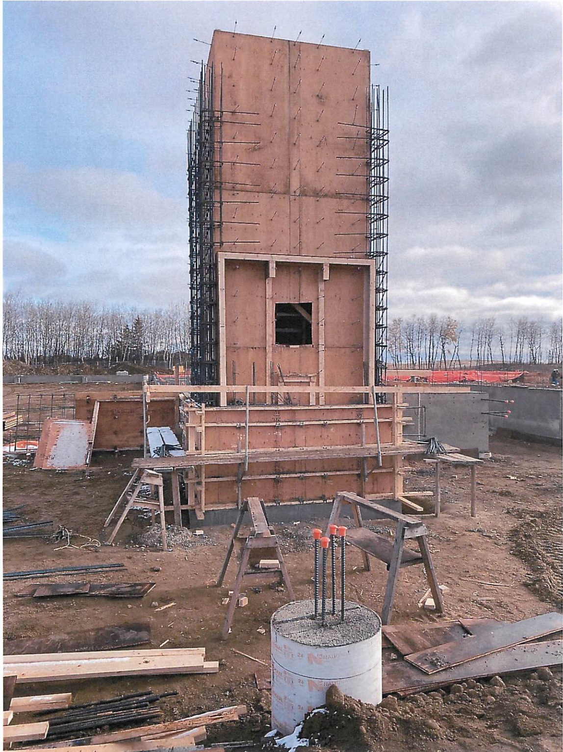
Elevator shaft formwork and reinforcement:
