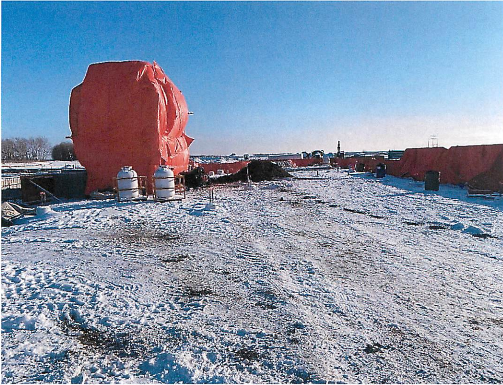
Lobby grade beams and elevator shaft:
