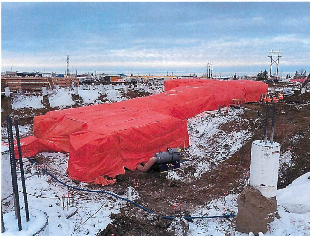
Hoarding for lap pool pipe installation:
