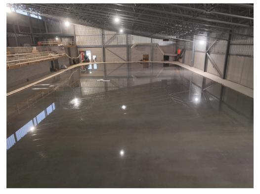
Figure 8 - South Arena - Slab with Water Cure
