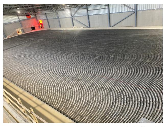
Figure 14- Arena South - Cooling Lines - Prepour
