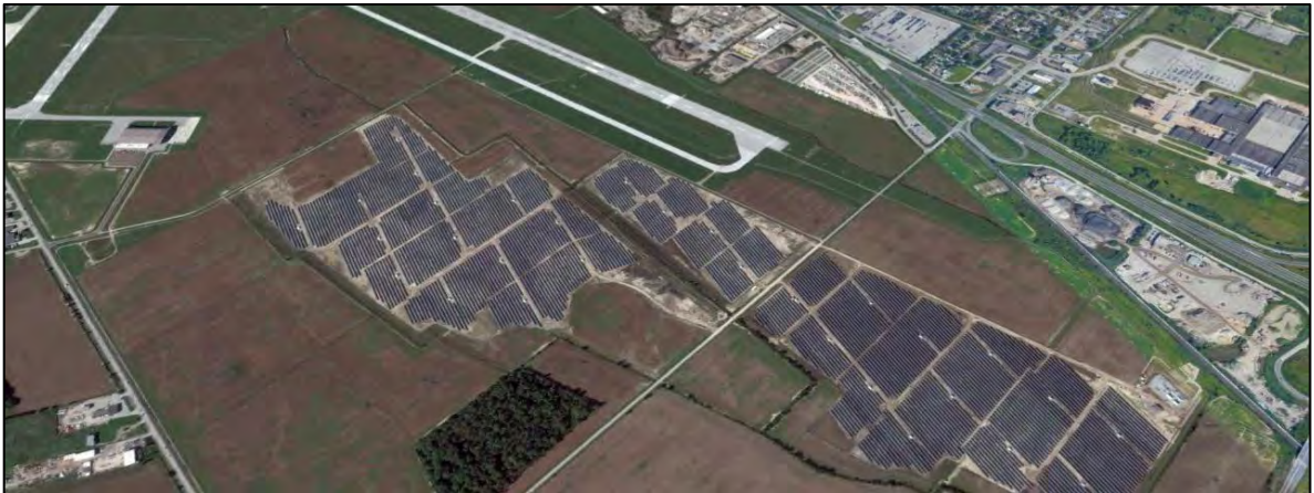
Photovoltaic generation facility at Windsor Airport (Google Earth)
