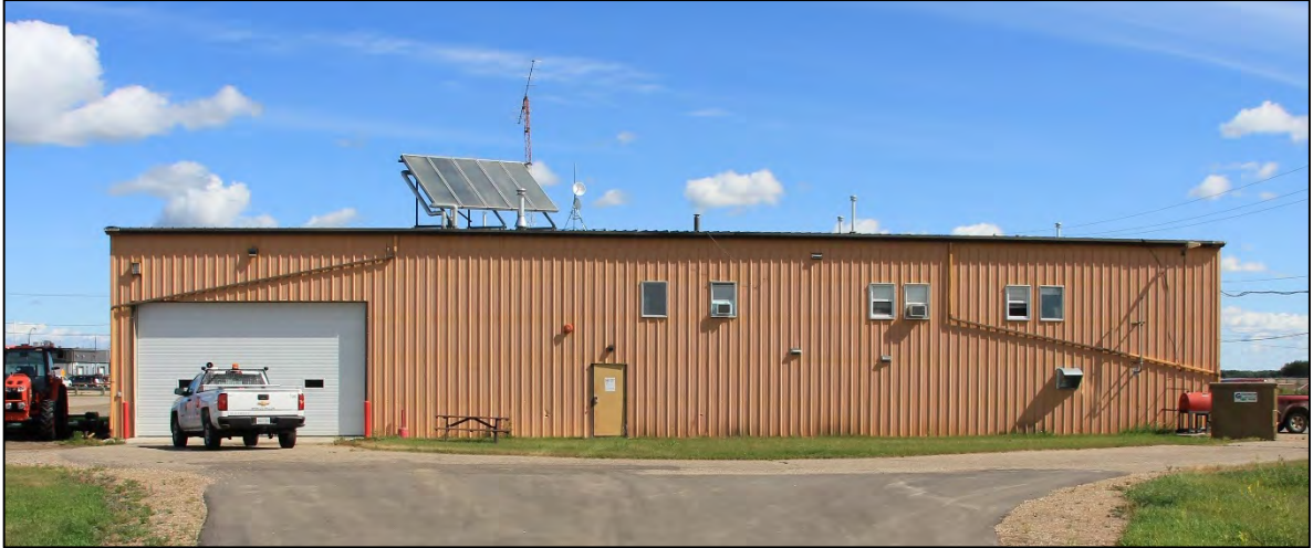
Airport maintenance building
