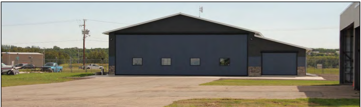
Existing airside hangar
